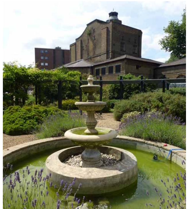
The surviving engine and pump house buildings © Rory Walsh
